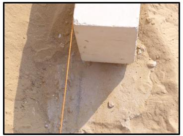
**Figure 17**. A patch of the gypsum-concrete foundations still preserving the original builder's ink guide line. A layer of sand is being used to cover it but, for the moment, the line is exposed to allow the modern builder's line exactly to follow it.
