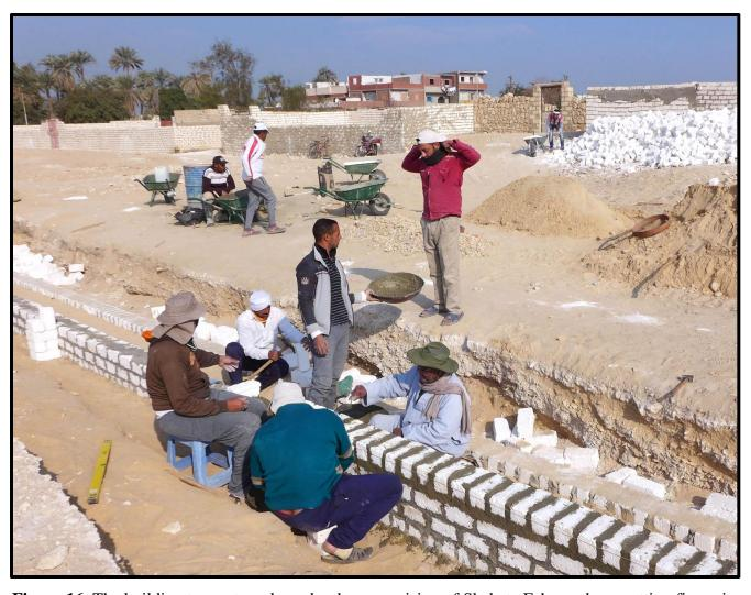
**Figure 16**. The building team at work, under the supervision of Shahata Fahmy, the squatting figure in the wide-brimmed green hat.
