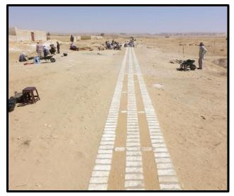
**Figure 19**. The foundations are made to be flush with the present surface of the desert. In the future they will be covered by a single course of blocks of fine Tura limestone cut to the ancient block size.
